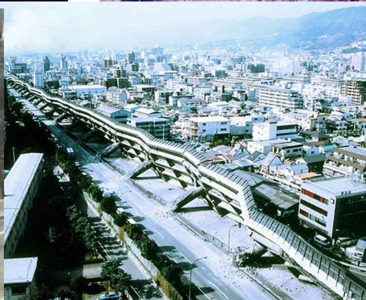
Collapsed Hanshin expressway in Kobe city
