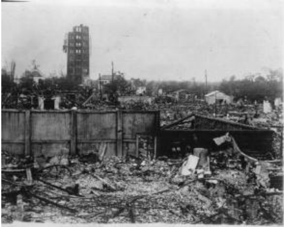
Collapsed Asakusa Ryo-Un Kaku
