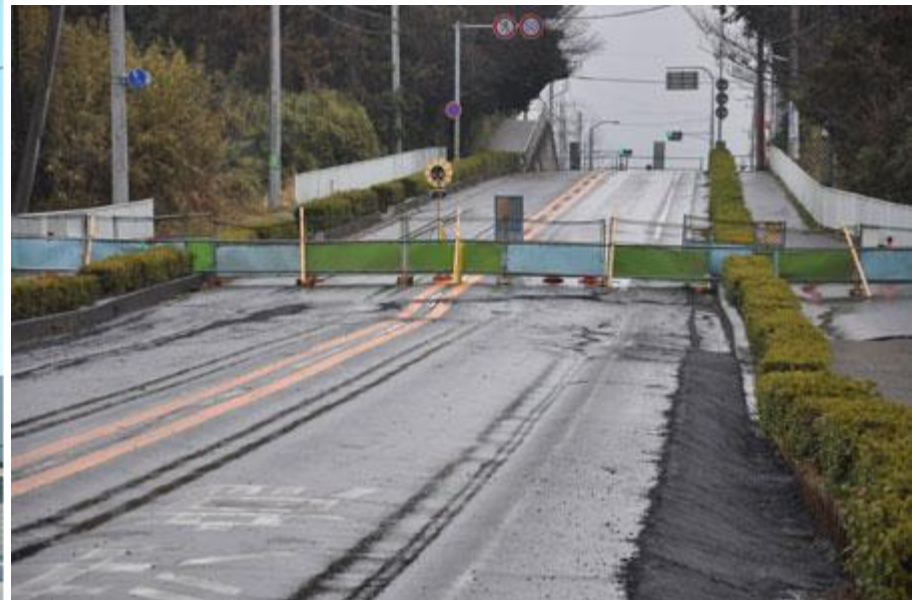
Closed road due to cracks near my home
