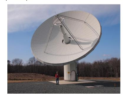
The analysis center is closely linked with the IVS Coordinating Center, the GSFC Technology Development Center, and the GGAO network station. GGAO is the home of the new 12 meter VLBI2010 antenna, GGAO12M, which recently participated in the first VLBI2010 broadband data taking sessions and is being used for
