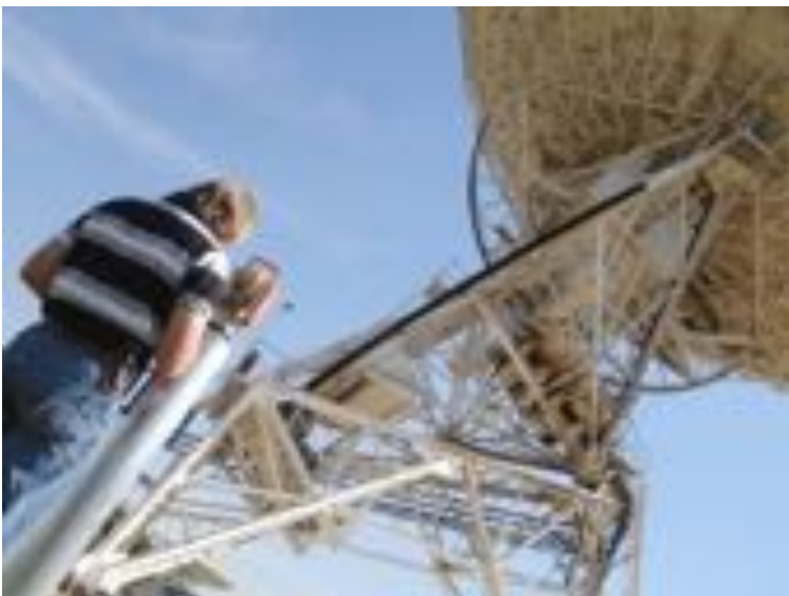
Fig. 2 Ludwig Combrinck surveying 26m polar shaft during 26m's bearing repair. Credit: Mike Gaylard
