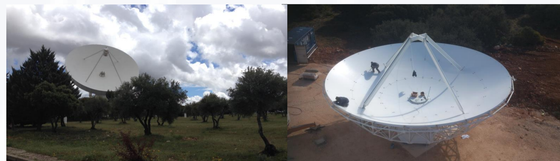
Figure 1. IGE VLBI infrastructure in Yebes: 40 m antenna (left) and parabola of the 13m antenna (right).
