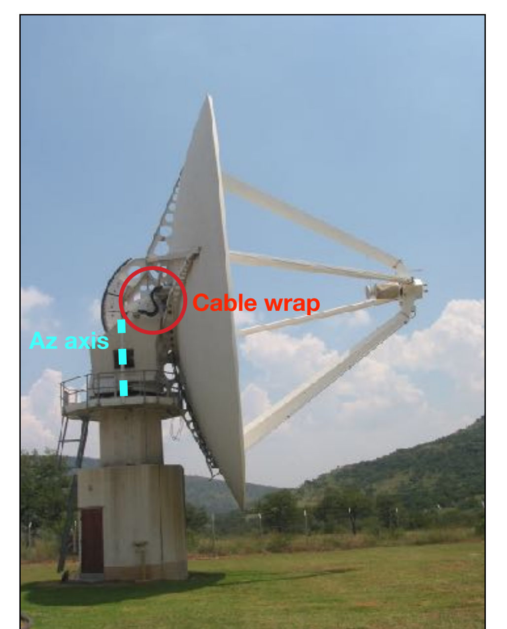
Figure 6: HartRAO 15-m - cable wrap obscuring one end of elevation shaft.
