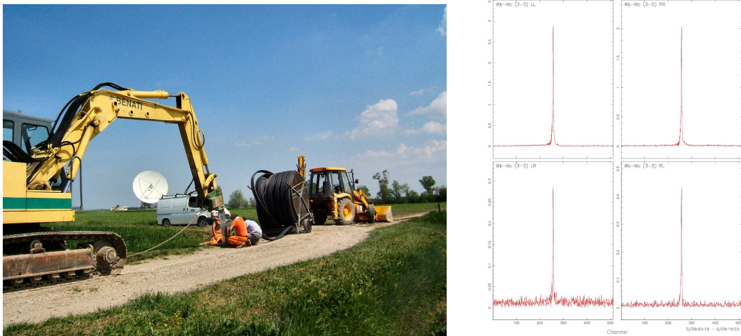
Figure 3: Left: Last-mile fiber works at the 32-meter radiotelescope in Medicina (Italy). Right: First real-time interference fringes (Mc-Wb).
