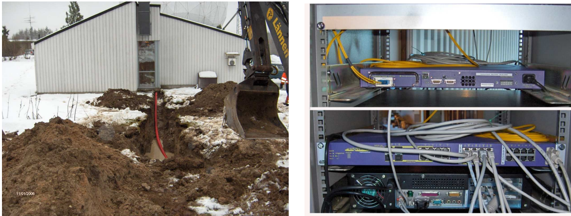
Figure 2: Last-mile fiber works (left) and equipment (right) at the 14-meter radiotelescope in Metsähovi (Finland).
