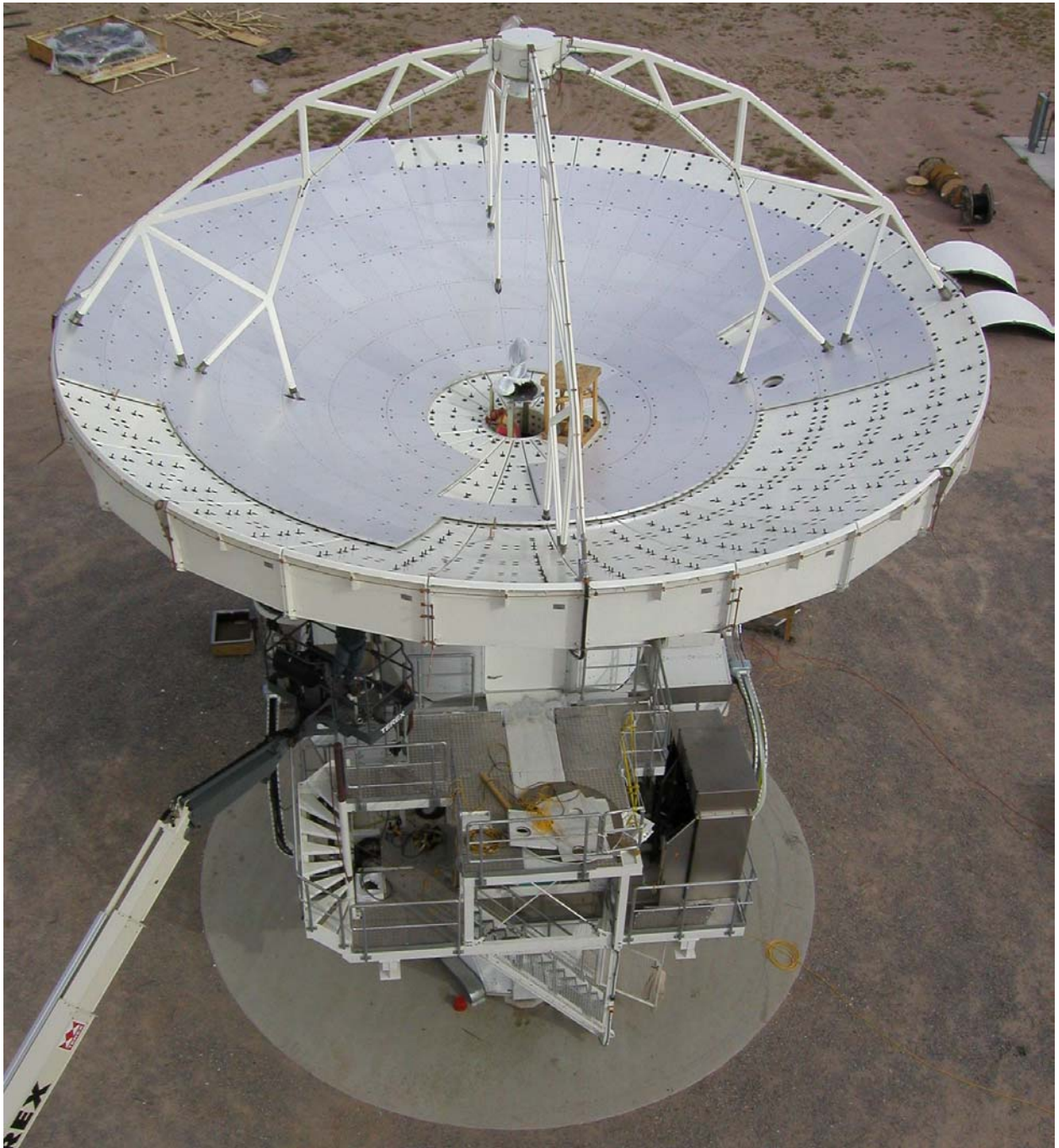
Figure 3. The antenna main structure erected showing current status of panel installation.
