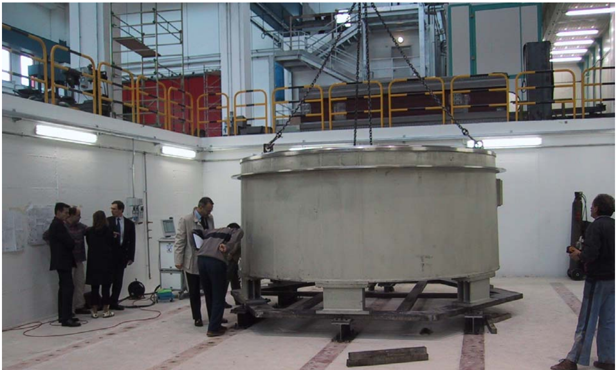
Figure 1. The AEC antenna pedestal being installed on test foundation connection.
