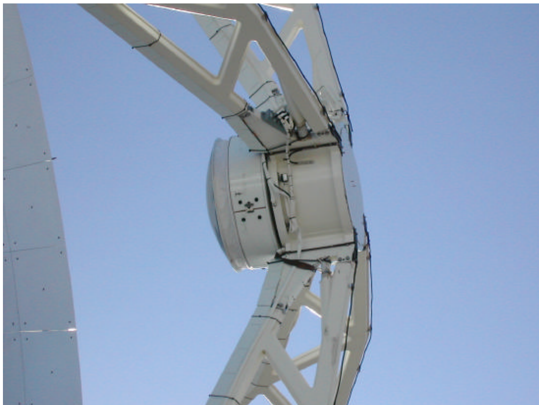
Figure 2.3.4 a: Nutating mounted on the VertexRSI antenna.
