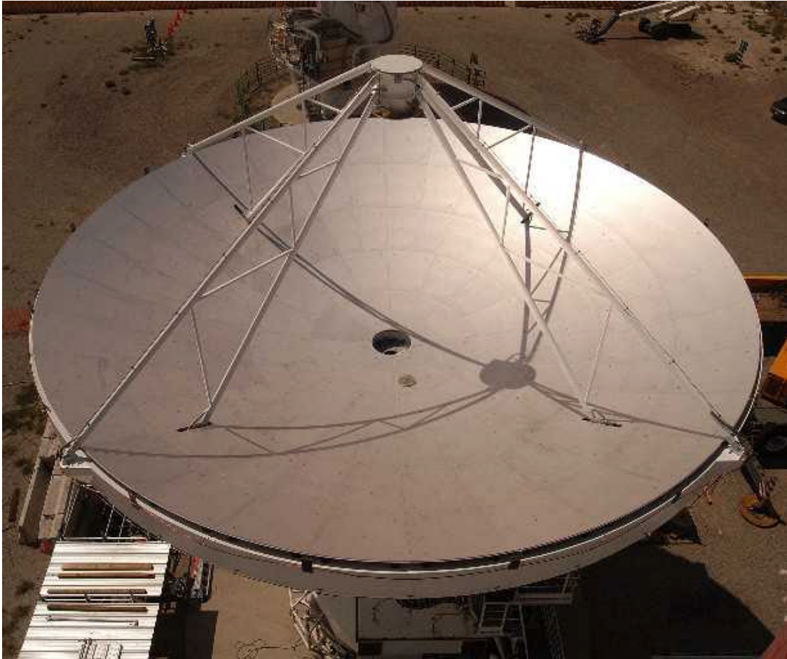
Figure 2.3.2 b: Main reflector and apex structure of the AEC antenna
