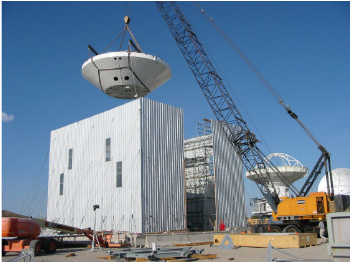
Fig. 2.3.2.a: The BUS being installed on the antenna
