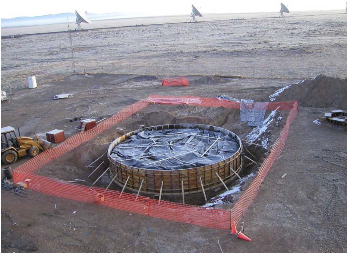
Figure 9. The AEC foundation as of December 6, 2002.
