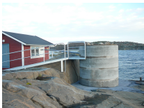
The tide-gauge well with pneumatic and radar-based sensors.
