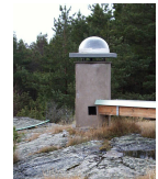
The ONSA GNSS site.
