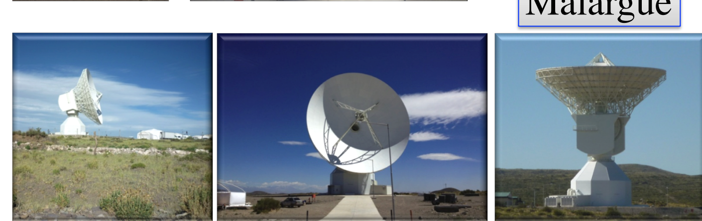
Fig. 2 ESA's 35-meter beam waveguide antenna, DSA03, Malargüe, Argentina. This dry site is at about 1500 meters altitude in desert behind the Andes mountain range (photo: L.A. White, 2012 Dec).
